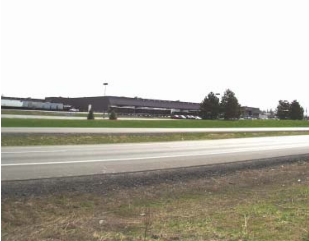
United Parcel Service Regional Distribution Center on Northern Boulevard
