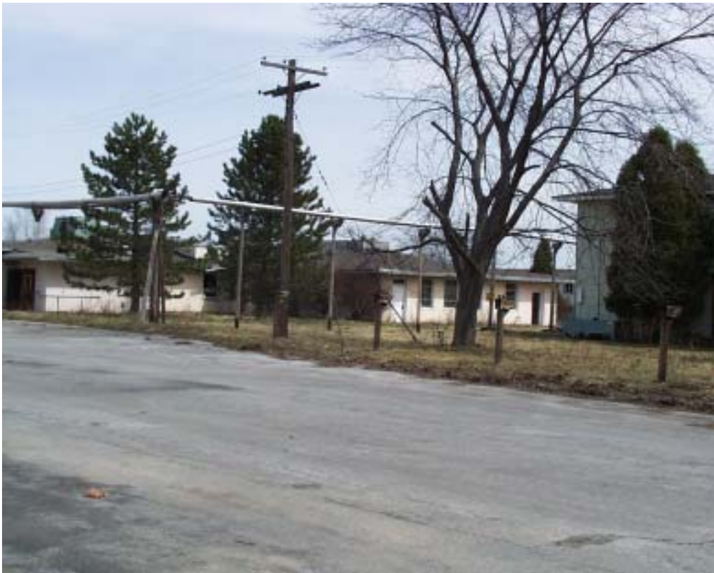
Former military housing and utilities on Hancock Air Park site
