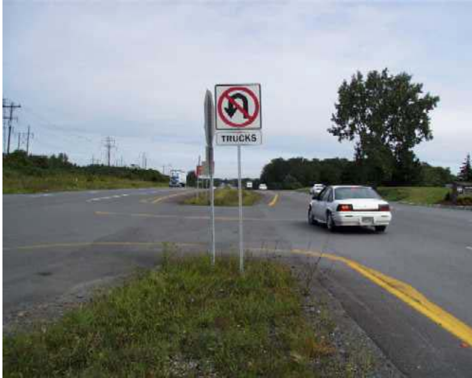
Sign banning truck turns in median on Northern Boulevard
