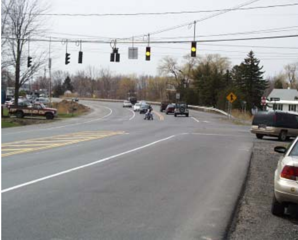
State Route 298 at Northern Boulevard looking east
